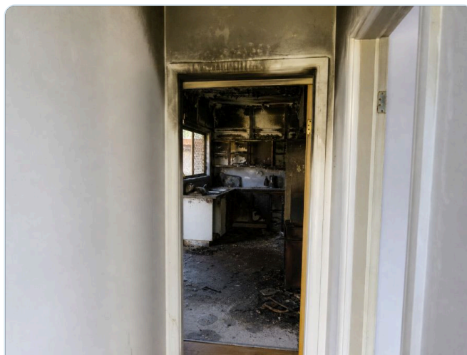
Photo 4 — Doorway transition to kitchen
